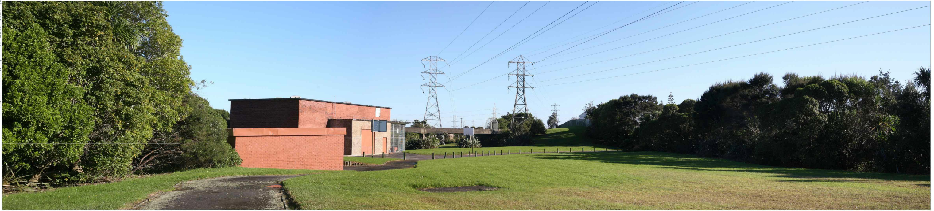
Existing View (from Walkway to East of Pump Station)
