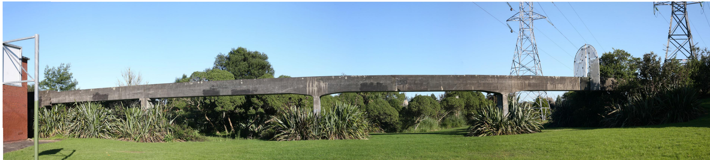
View to West from carpark in front of existing Pump Station
